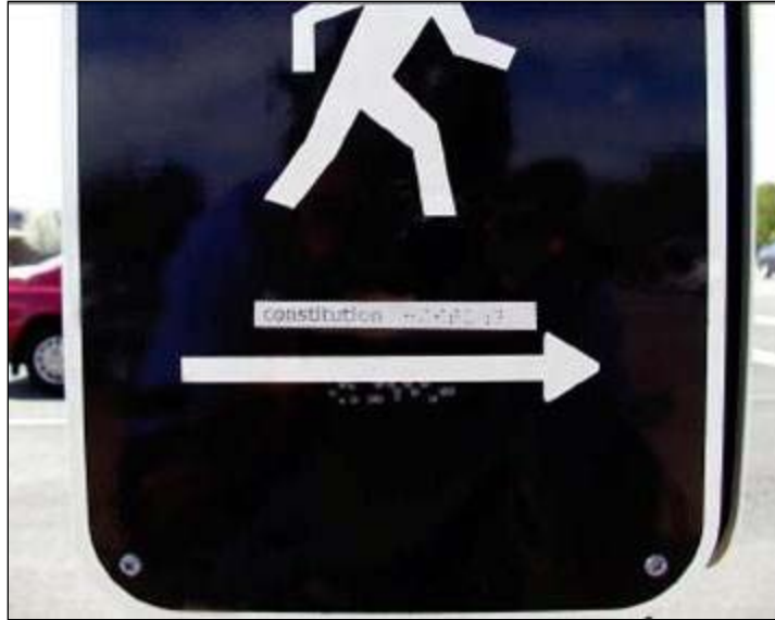
Figure 14: Braille sign installed backwards, with manufacturers' label showing. Label includes street name and print of how Braille should look. Braille beneath arrow is backwards version of the print version shown on label and is indented, rather than raised.
