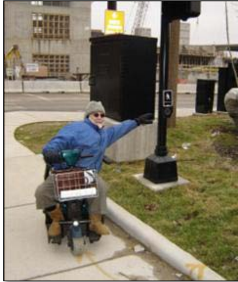
Figure 12: In this new construction, APS is located too far from the sidewalk to be reached by a user of a wheelchair or scooter.
