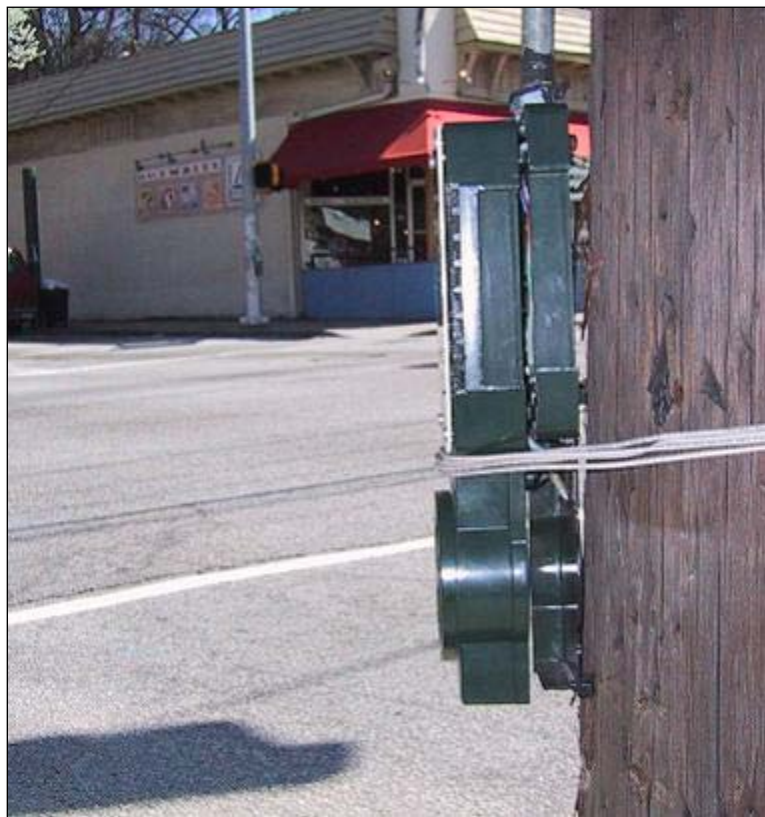
Figure 11: APS that was damaged in a crash and temporarily reinstated with wire.
