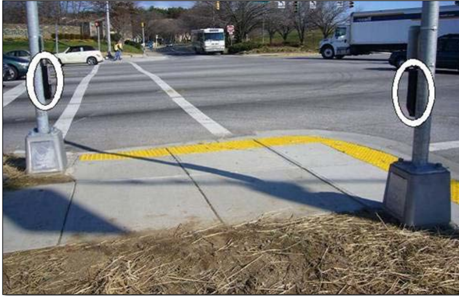
Figure 4: Installation of APS on two separated poles, aligned with crosswalk lines (APS devices circled)
