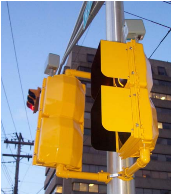
FIGURE 8 (LEFT): NOVAX DS 2000 SPEAKERS MOUNTED ON TOP OF PEDHEADS
