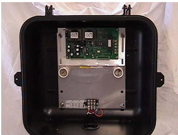
FIGURE 3: CAMPBELL CONTROL UNIT INSTALLED A 16 INCH PEDHEAD.
