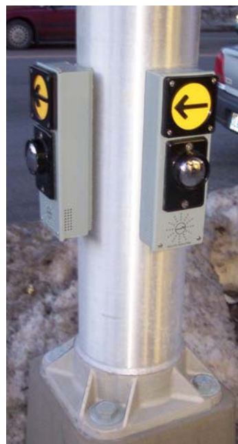
FIGURE 8 (LEFT): NOVAX DS 2000 SPEAKERS MOUNTED ON TOP OF PEDHEADS
