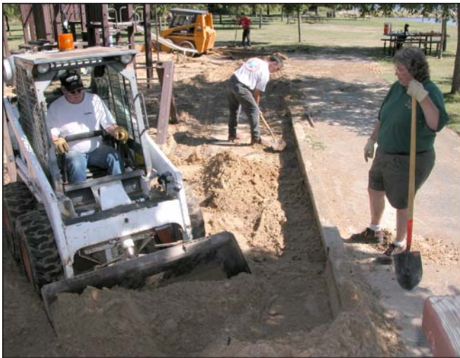
Figure 2—Removal of sand from existing playground surface.
