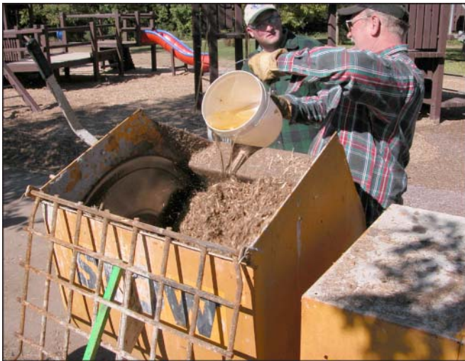
Figure 6—Mixing of binder and EWF in mortar mixer.
