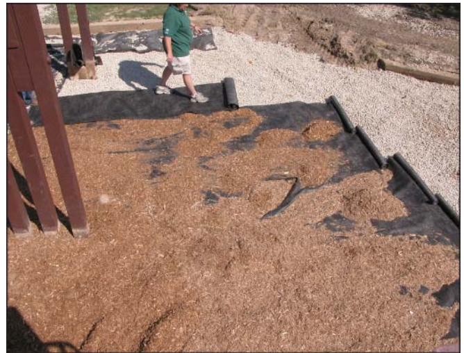
Figure 4—Completion of drainage system; second layer of fabric laid over drainage rock.
