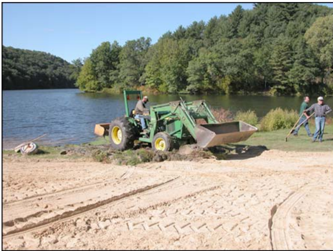
Figure 2—Grading of beach path to waterline.
