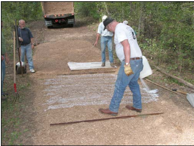
Figure 11—Treatment of wide bridle trail (site 2): spray application of Vitri-Turf in background and drip-bucket application of Soil-Sement in foreground. Note use of polyethylene-covered plywood for compaction and leveling of Vitri-Turf SEWF.
